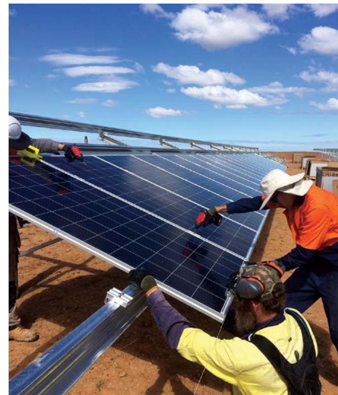
GOLDEN GROVE INSTALLATION OF 3,700 PV PANELS ON 6,000m 2 OF LAND
