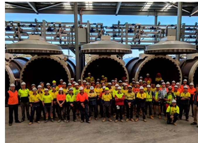
THE HEBEL TEAM AT HEBEL'S AUTOCLAVED AERATED CONCRETE PLANT UNDER CONSTRUCTION IN SOMERSBY, NSW
