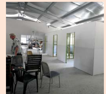
GYPROCK PLASTERBOARD INSTALLATION, TIN CAN BAY MENS' SHED
