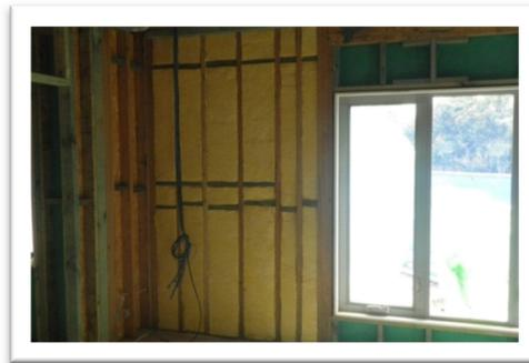
2. Where electrical cables penetrate the lining, the insulation should not be dislodged or be deformed to create air gaps.
