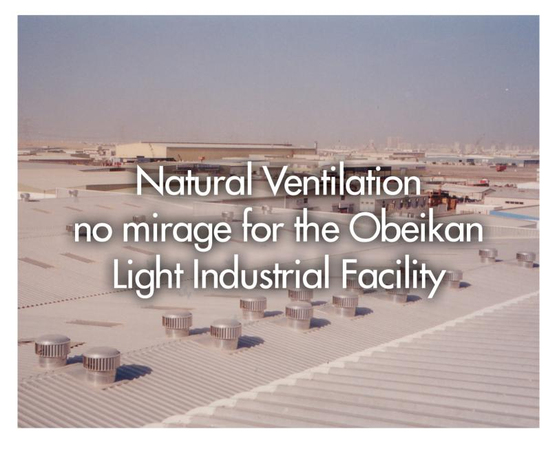
For over 25 years, the robust Hurricane® range of Vertical Vane™ natural ventilation technology has been built to endure tough climatic conditions and the harshest operating environments – just like the sand storms that occur in the hot desert environment of the Red Sea coast.
