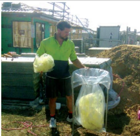
Monier in Victoria has developed an innovative solution with a major customer to recycle the plastic stretch wrap that is used to transport roof tiles to building sites. The Monier team designed a unique bag collection system in which the wrap is collected and transported away from the site for recycling. Monier has rolled out the system extensively throughout Victoria.
